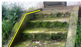
Figure 9. Obtuse angle in barrier
