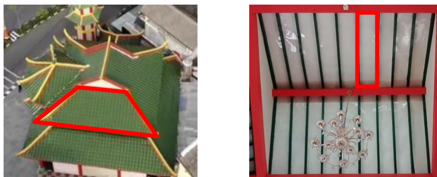
Figure 2. (a) The Roof form Outside, (b) The Roof form Inside
